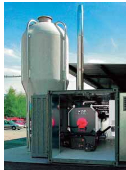
Containerized boiler package (pellet silo field supplied)
